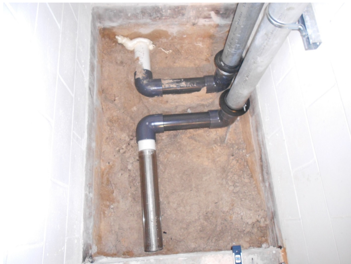
Figure 3. Photo showing system piping prior to backfilling.
